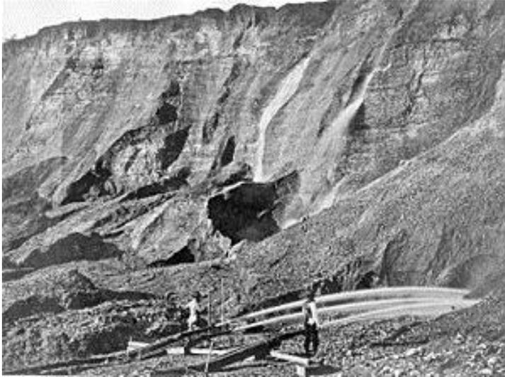
Hydraulic mining uses high pressure jets of water directed through a giant nozzle, called a "monitor," at gold-bearing hillsides. The extremely high pressure stream washed entire hillsides through enormous sluices to recover the gold. This technique was devastating to the environment and was outlawed in California in 1884.
