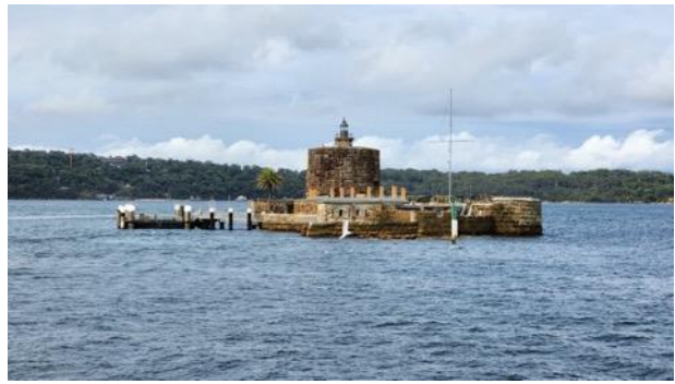
Photo 5: Fort Denison, Sydney Harbour, Australia
