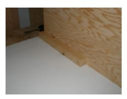
Using my IKEA-sense of how these things should go together, I started with the bottom panel of the booth and attached the 1¾" x 1¾" runs of supports along the inside of the booth, leaving room for the thick sides to be attached and the back panel to be attached later.
