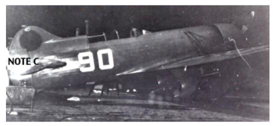
C-1935 Bendix: Colors/markings as B above except the MacRobertson race number was crudely painted out with a slightly darker green than was the original and race number "90" was applied to the fuselage in white. Landing lights and drift window were deleted. The landing light holes were plated over with shaped, bare-aluminum patches.
